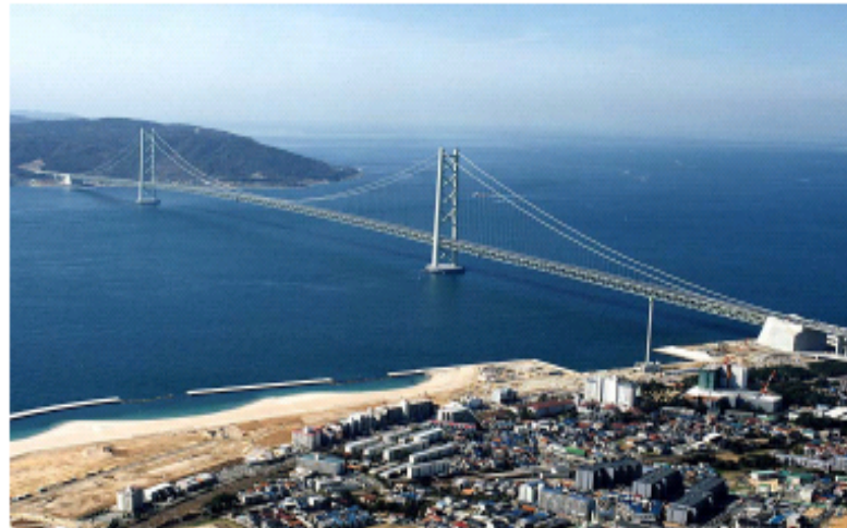
Akashi Bridge suspension bridge In Japan
